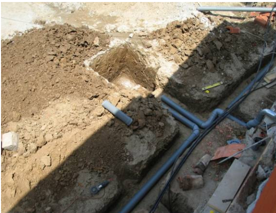
the water installation around the toilets is being installed and the main property sewage is dug up as you see on the above right photo.
