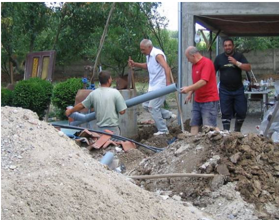
The plumber team working hard connecting the toilets to the main property sewage.
