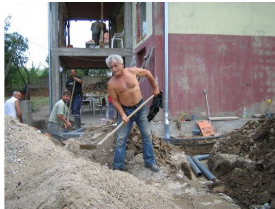
the water installation around the toilets is being installed and the main property sewage is dug up as you see on the above right photo.
