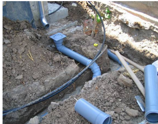
The plumber team working hard connecting the toilets to the main property sewage.
