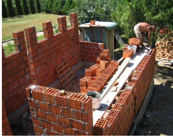
the walls of the toilets are rising fast.
